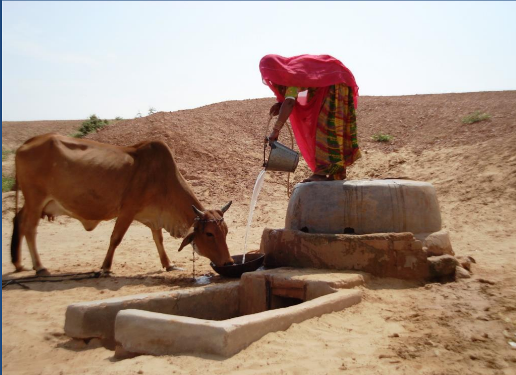
Woman fetching water from renovated beri . Beri's mouth is covered with a concrete platform.
