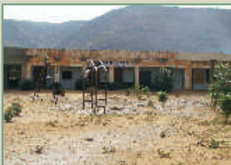
Notki School before intervention
