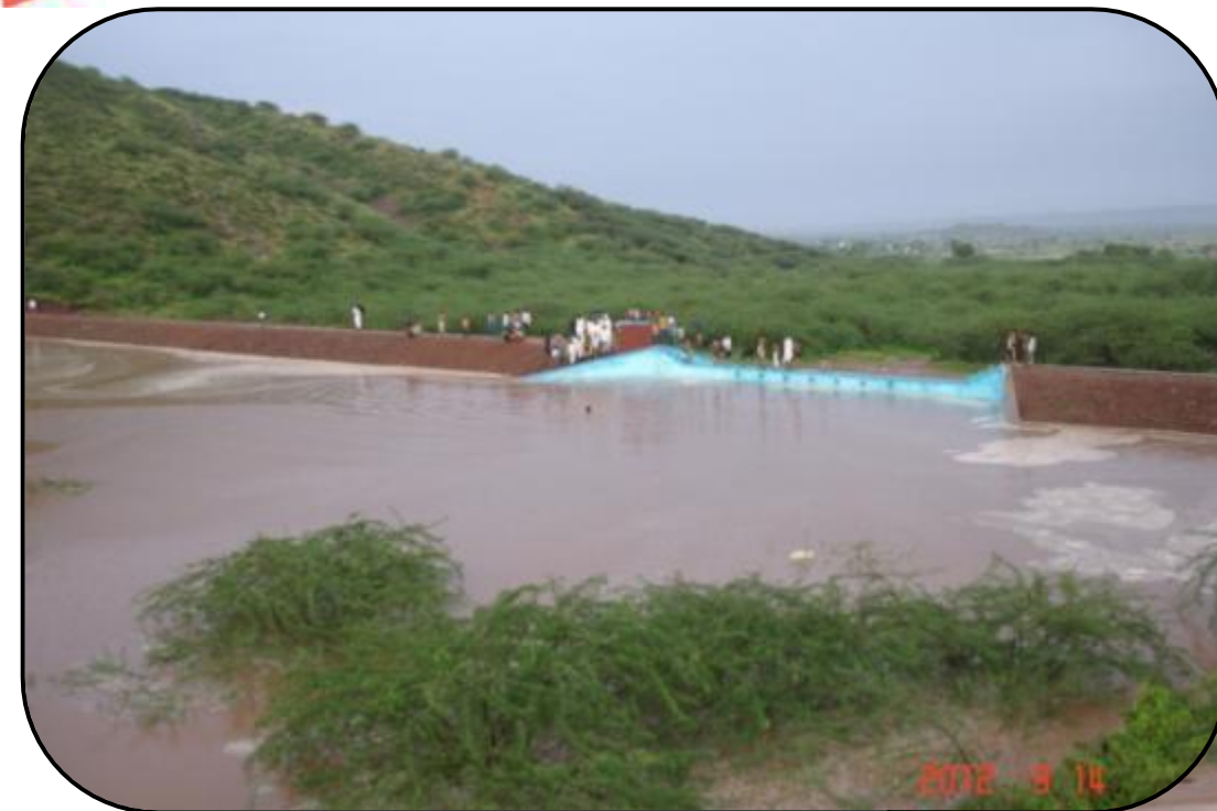
Check dam full with rainwater in Patkhori village
