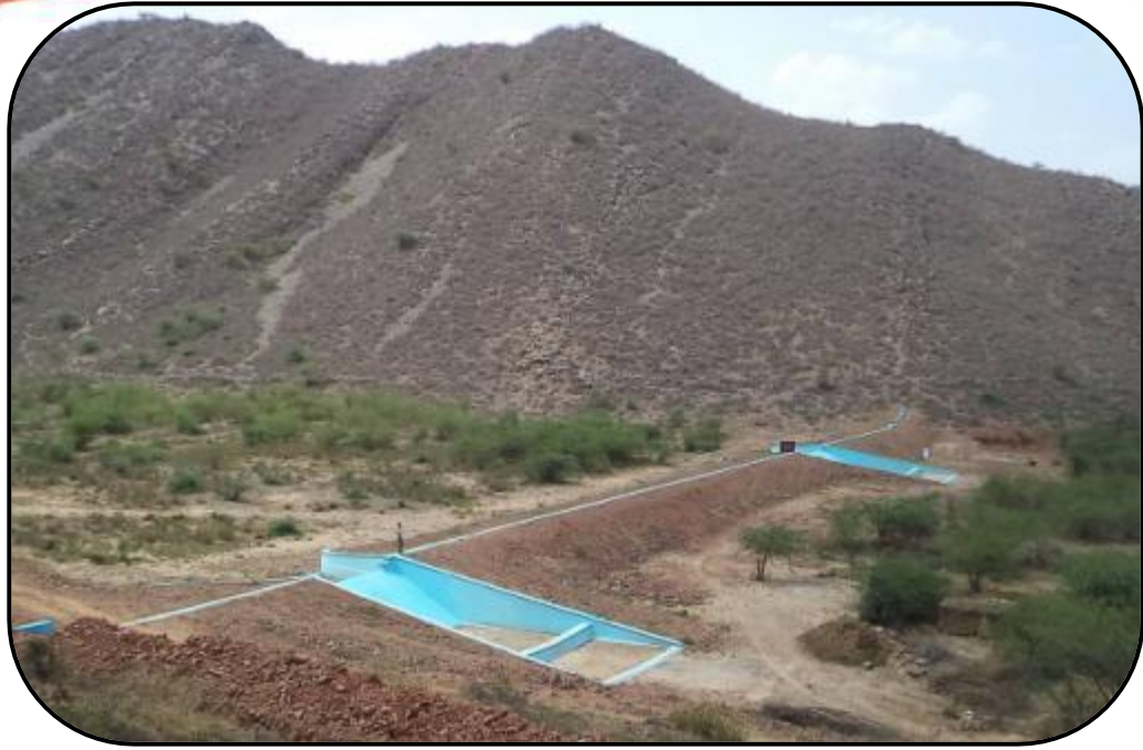
Another check dam in Rawli village supported by Japan Embassy
